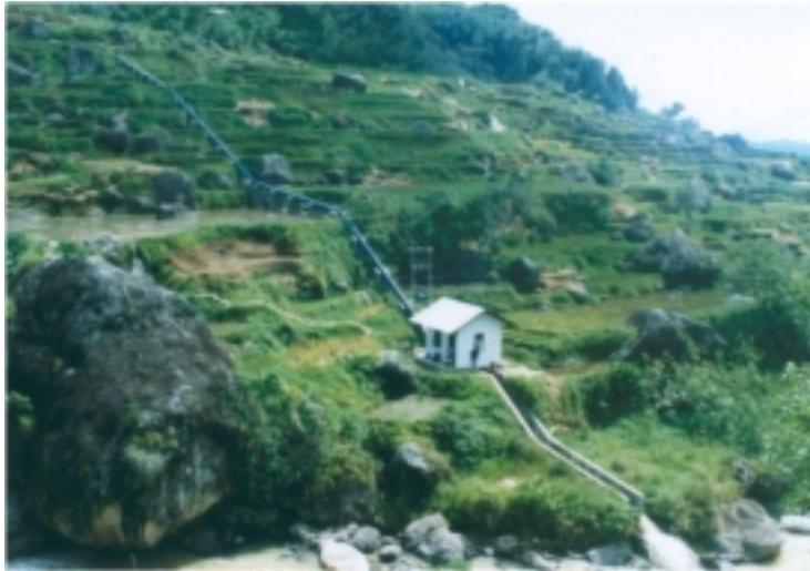
**Micro-Hydro-Plant (MHP) Taba – Powerhouse, headrace and penstock**
